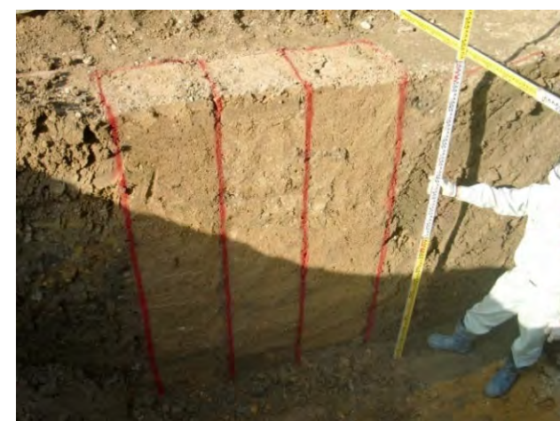
遮水壁断面確認
